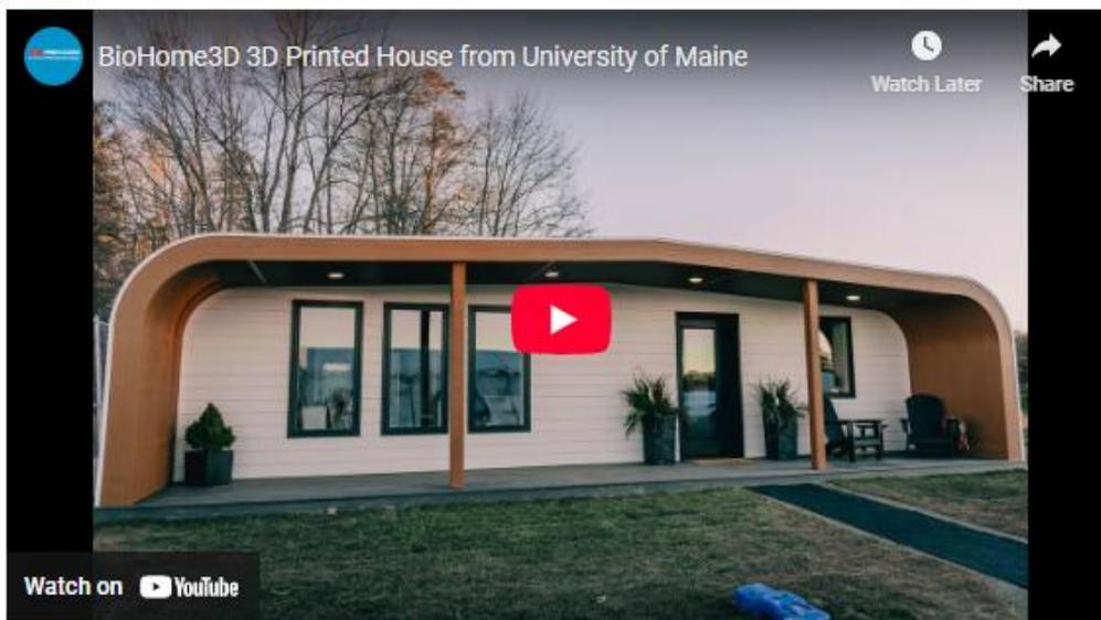
BioHome3D is a 3D-printed house constructed out of 100 percent bio-based materials. | Video: 3DPrint.com
